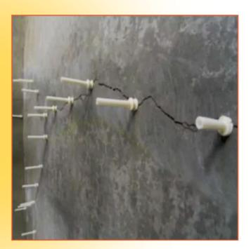
**DESCRIPTION:** Shoolin EIG is two port, Solvent free, Low Viscosity epoxy resin System is mixed in the Proportions Supplied to farm a Strong Permanent bond and seal in cracks in concrete and masonry this product is designed to be injected into Cracks using Suitable resin injection equipment.
